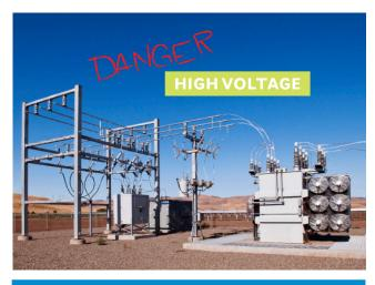
Between the generating station and consumer, electric power may flow through several substations at different voltage levels. A substation may include transformers to change voltage levels between high transmission voltages and lower distribution voltages, or at the interconnection of two different transmission voltages.
