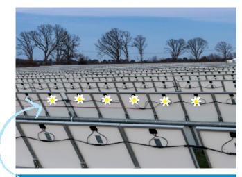
The electric current that's created is captured through nodes and wiring in the panels. Individual panels are connected, like a daisy chain, by string wire to make up a row.
