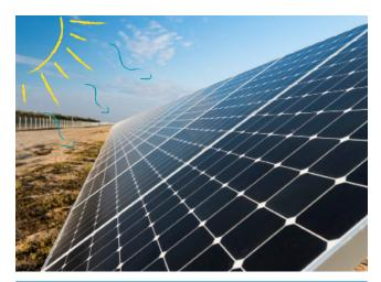
The sun's rays are absorbed by the photovoltaic cells of the panels. When the sun's rays interact with the silicon cell, electrons begin to move and this created a flow of electric current. The electricity created is DC or direct current.
