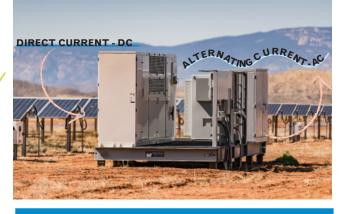
The combiner boxes feed the consolidated DC energy through underground cables to an inverter. The inverters convert the direct current (DC) to alternating current (AC), which allows us to use the energy from the sun! The number of inverters on a single solar site depends on the overall size and megawatts produced.
