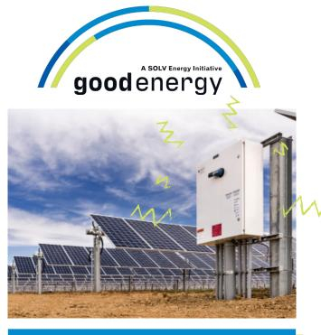
These rows of panels feed into a combiner box, which are set up at the end of the row. The amount of rows per combiner box is all dependent on the size of the individual rows. The job of the combiner box is to consolidate the DC power.
